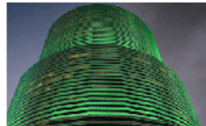
Bank of America Tower
